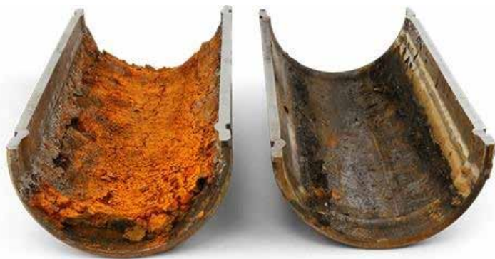
Corrosion of internal surface elements of oil pipelines
